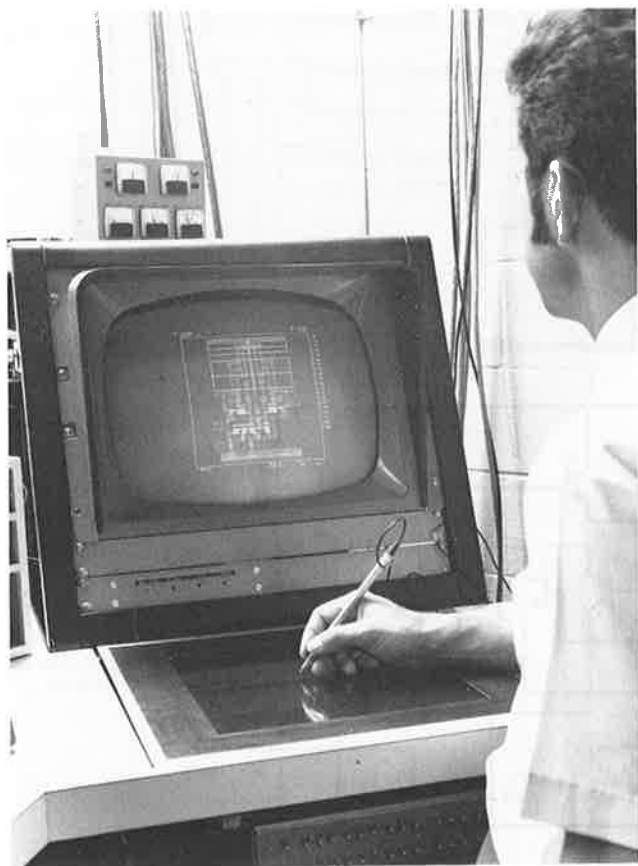
Fig. 8.44 Mask making using the TX-2 computer and an interactive tablet-scope drafting program.
